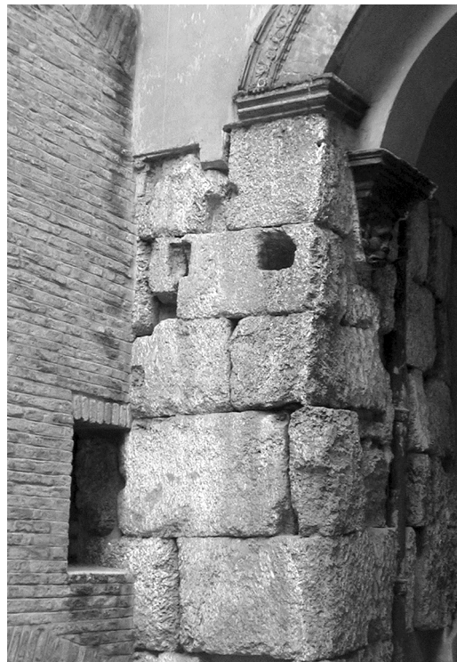
Fig. 1 – Remnants of the IV-VIII century AD selenite walls, preserved and recycled in the Ghisilardi Fava Palace at Bologna .
