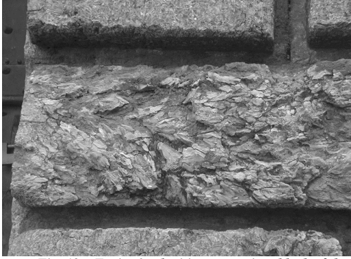
Fig. 12 – Facies 3 selenitic gypsum in a block of the Garisenda tower of Bologna.
